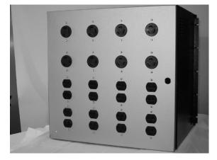
**Output circuit breaker(s) and/or panel boards** with ground and neutral provisions are provided inside the unit for connecting receptacle, hard wired, and external load(s) as required.
